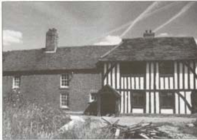
1994 - unauthorised alterations in progress
