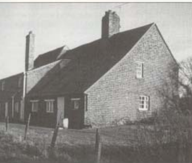
Old Hall Farm, north west elevation, March 1991
